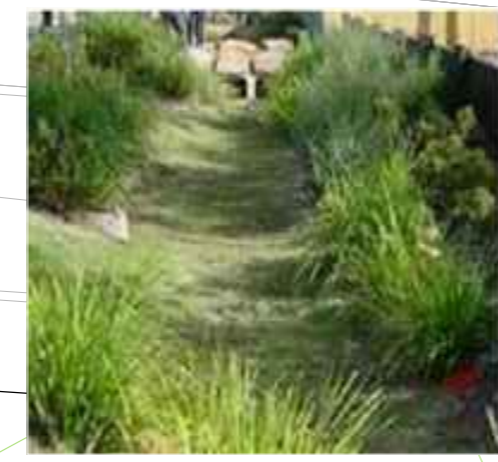
Linear Dry Swale Bio Detention No standing water
